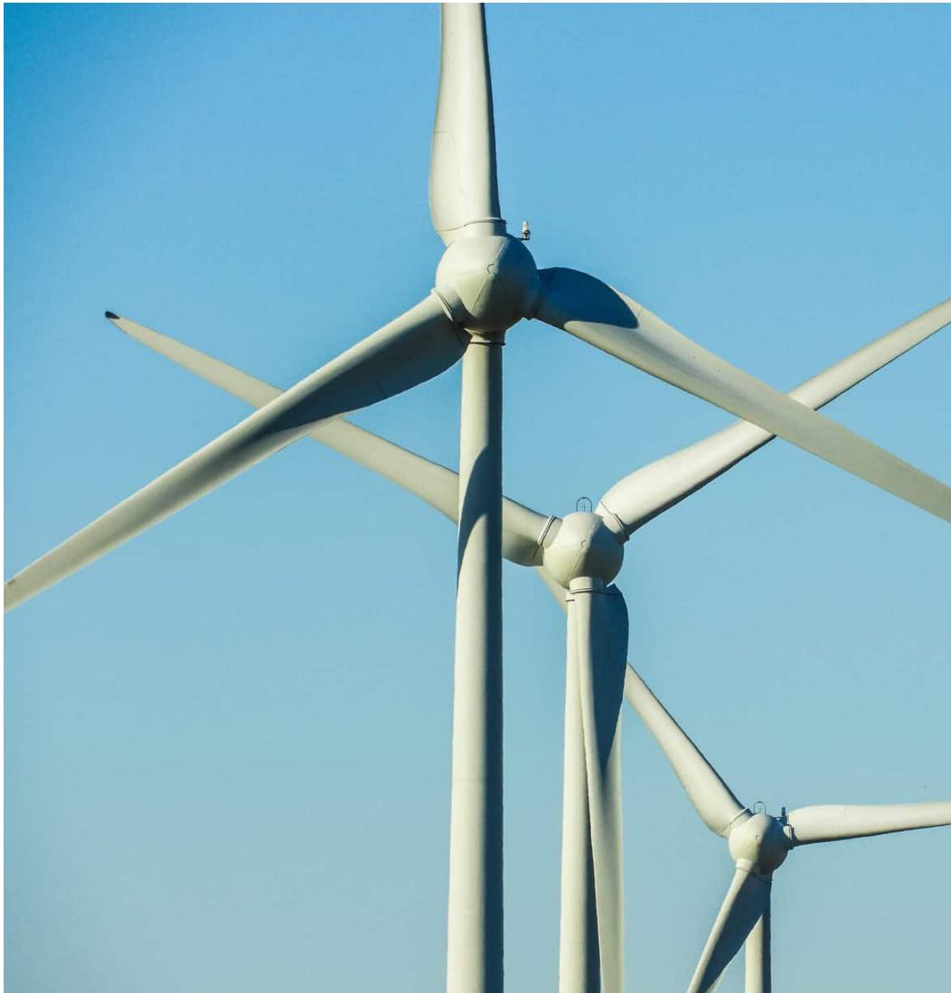
Wind turbines on Utah's trust lands.
